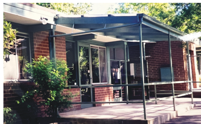
The old EPC Building
